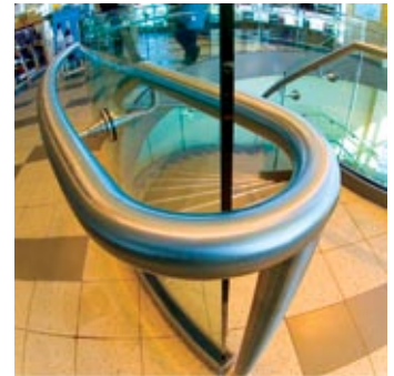
Stainless steel rolled and formed railing detail
