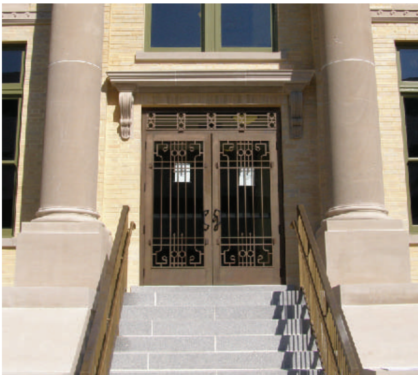
Exterior entrance doors and railings.
