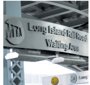
Waterjet cut stainless steel letters pin mounted with stand-off
