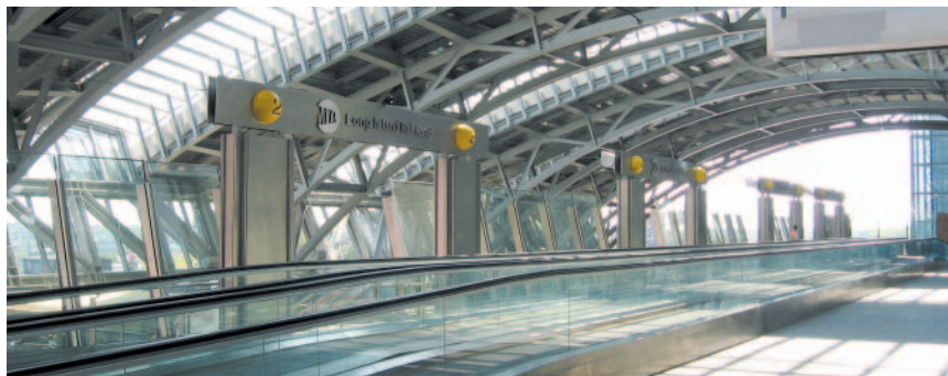
Array of girders spanning approximately 150 feet
