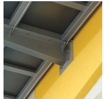
(31) outriggers connected to building column
