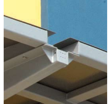
Eavestrough detail, prior to final cladding
